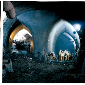
Figure 1.5 Pilot & enlargement construction sequence
