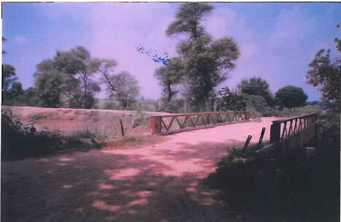
Figure 5.2: An unlined canal.
