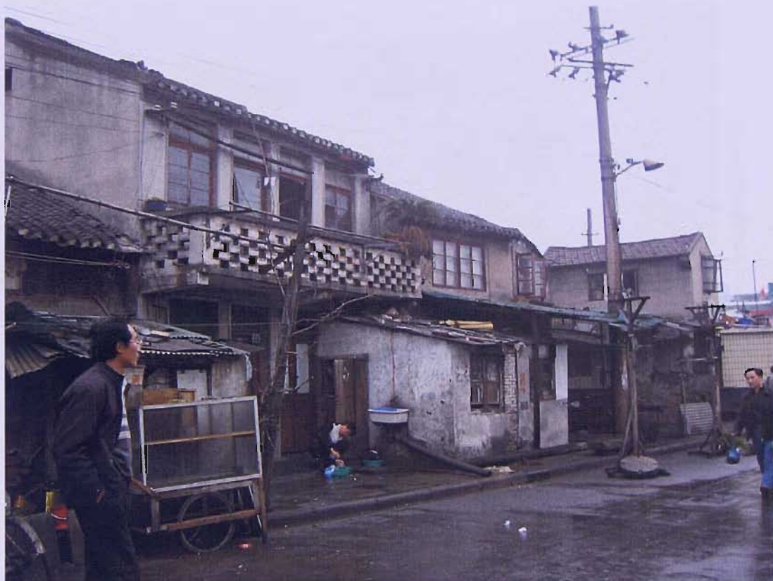
A: Dilapidated low-rise houses in SJZ
