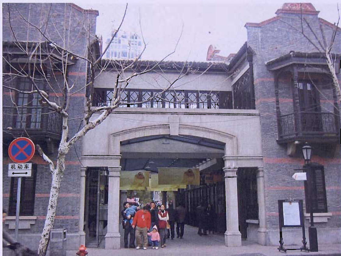
D: The refurbished doorway of lilong houses
