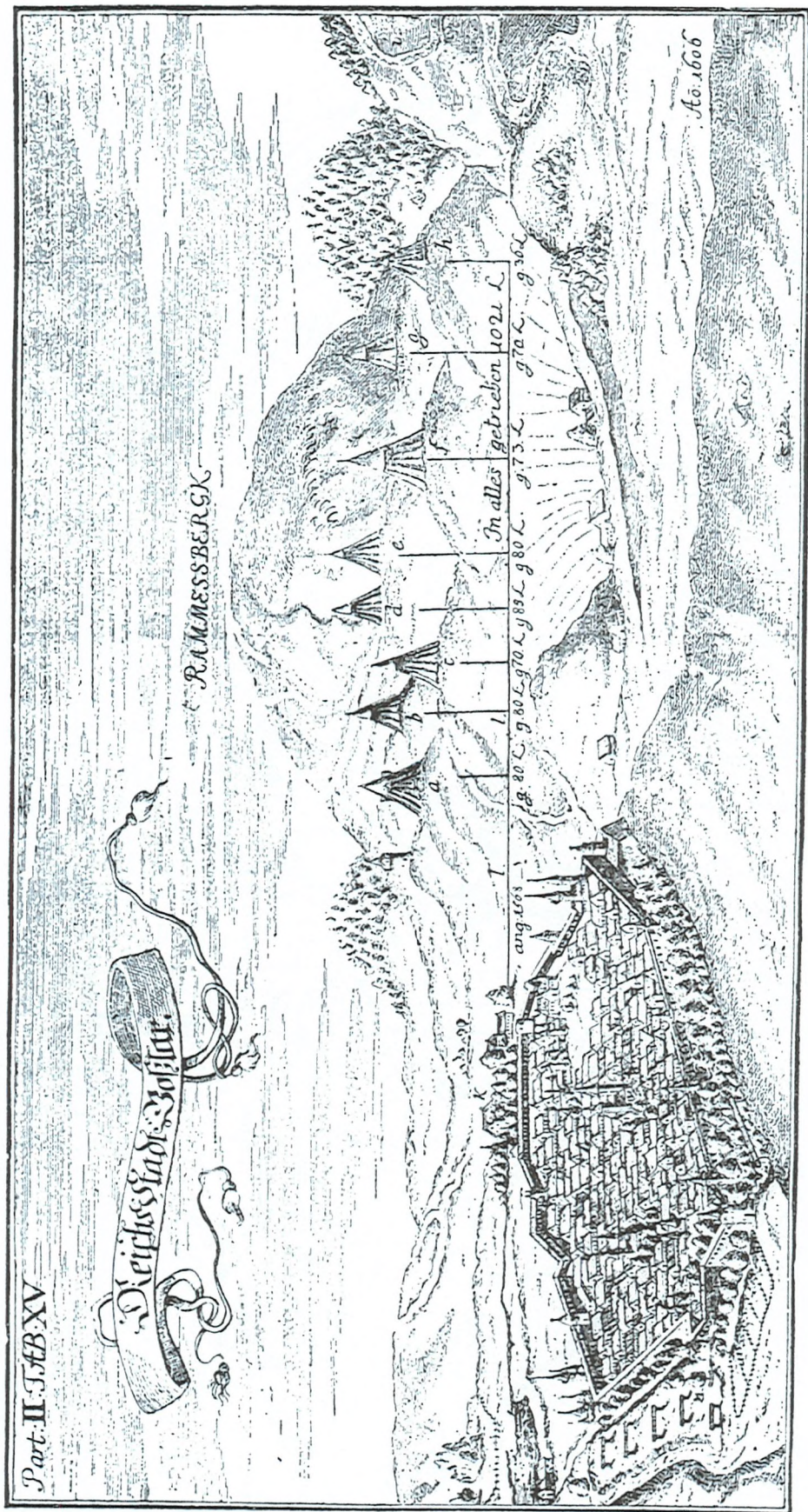
Fig. 14 A copy of a copperplate engraving by Daniel Lindemeyer c. 1606. The out-of-scale drawings of the tent-like shaft covers and the marking of the drainage tunnels were used to explain the mining installations at the Rammelsberg.
