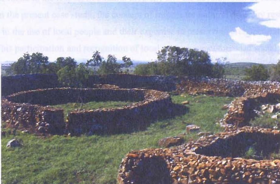
Figure 51: Thimlich Ohinga walls after restoration (Joffroy 2005: 102).
