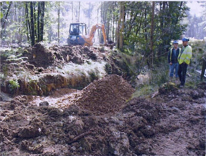
Figure 4.14 Channel infilling during restoration at the Restored site.
