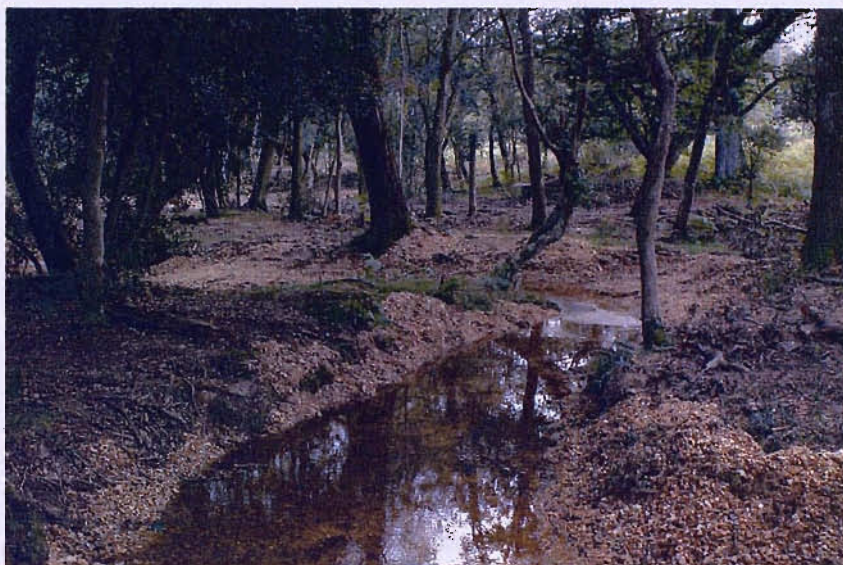
Figure 6.10 New gravels with fines that were used to infill over-deepened channels.
