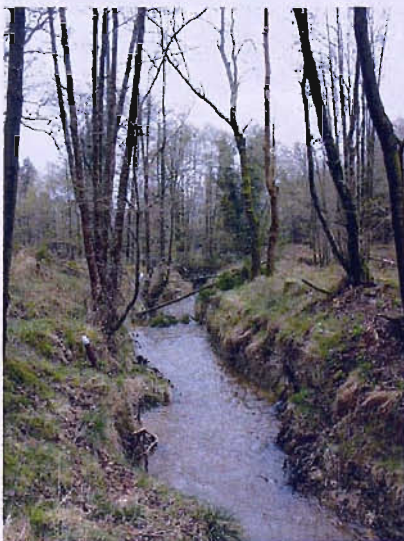
Figure 4.12 Restored site before restoration looking upstream. Note the straight, deep channel with spoil heaps on both sides.
