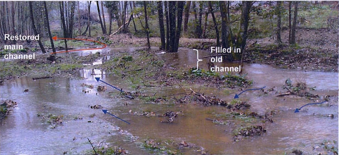
Figure 6.28 Flow from the filled-in channel depression spilling into floodplain channels and back into the main channel (Site 2) (blue arrows = floodplain flow; red arrow = main channel flow).
