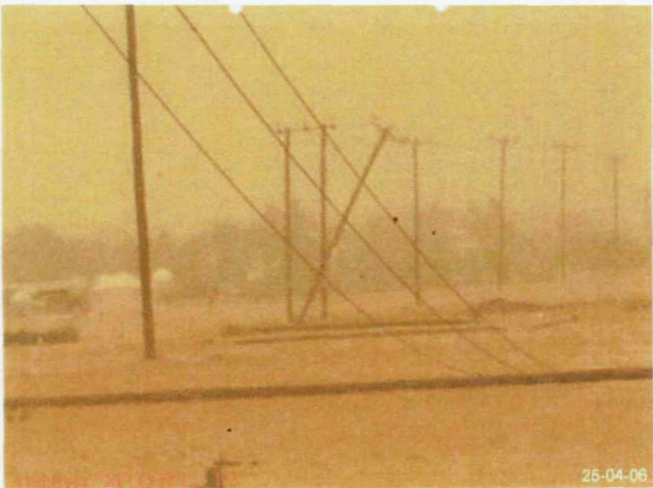
Figure 7.2 High Impedance Fault cases in Kuwait A, B, C, E, H- 11kV overhead line touching trees D, G – Fallen energized overhead line F – Black spots in the sand around the line due to arcing
