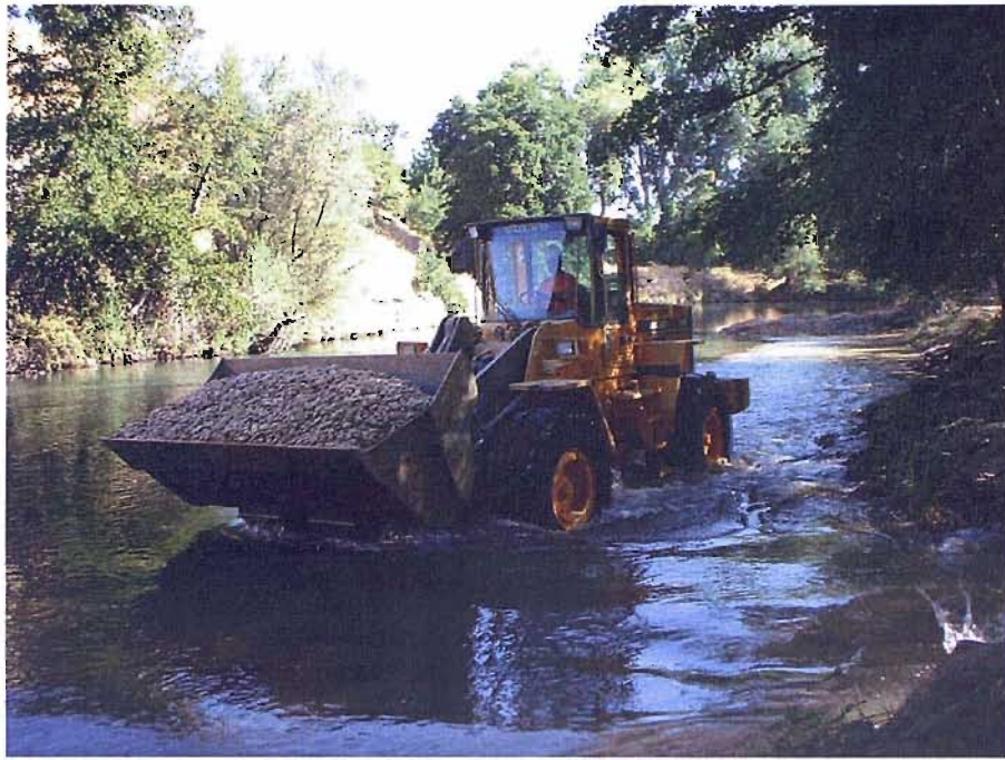
FIGURE 1.1: Despite all the rhetoric calling for 'catchment-scale restoration', most PHR involves active intervention (i.e. construction of habitat features) at the reach scale as shown here. In this case gravel is being placed in a channel downstream of a dam to construct riffle and bar habitats for salmon. Photo from PHR in 2001 on the Mokelumne River, California (photo by Author).
