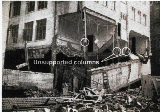
Fig. 1. 3 Bracing from panel walling (Baker, 1948)
