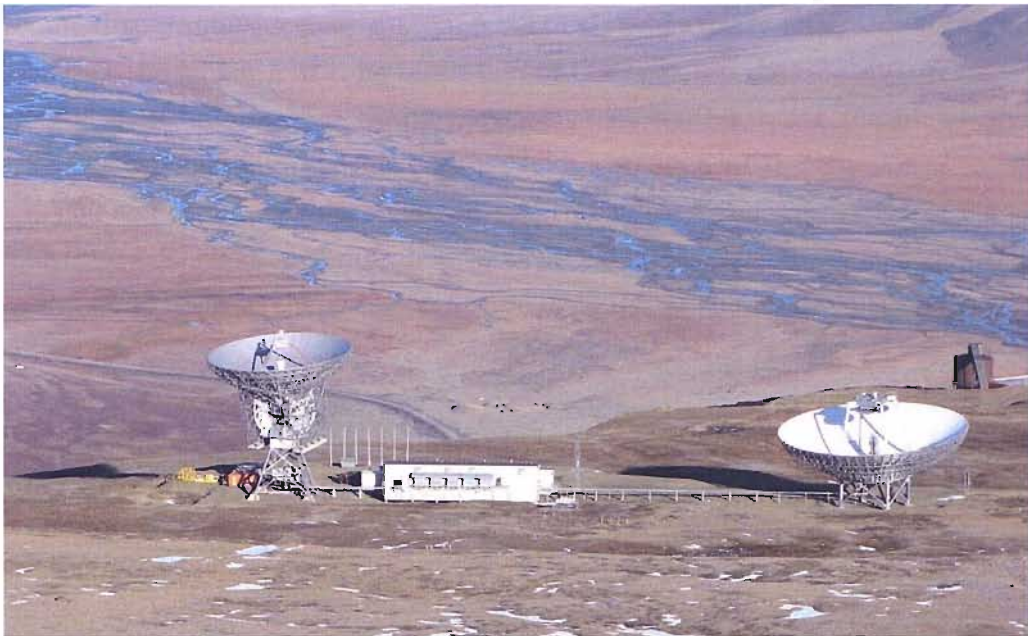
Figure 2.5: Photograph of the EISCAT Svalbard Radar, taken from further up the mountain of Breinosa on 6 September 2007. The 32 m dish is to the left of the photograph, and the 42 m dish is to the right.
