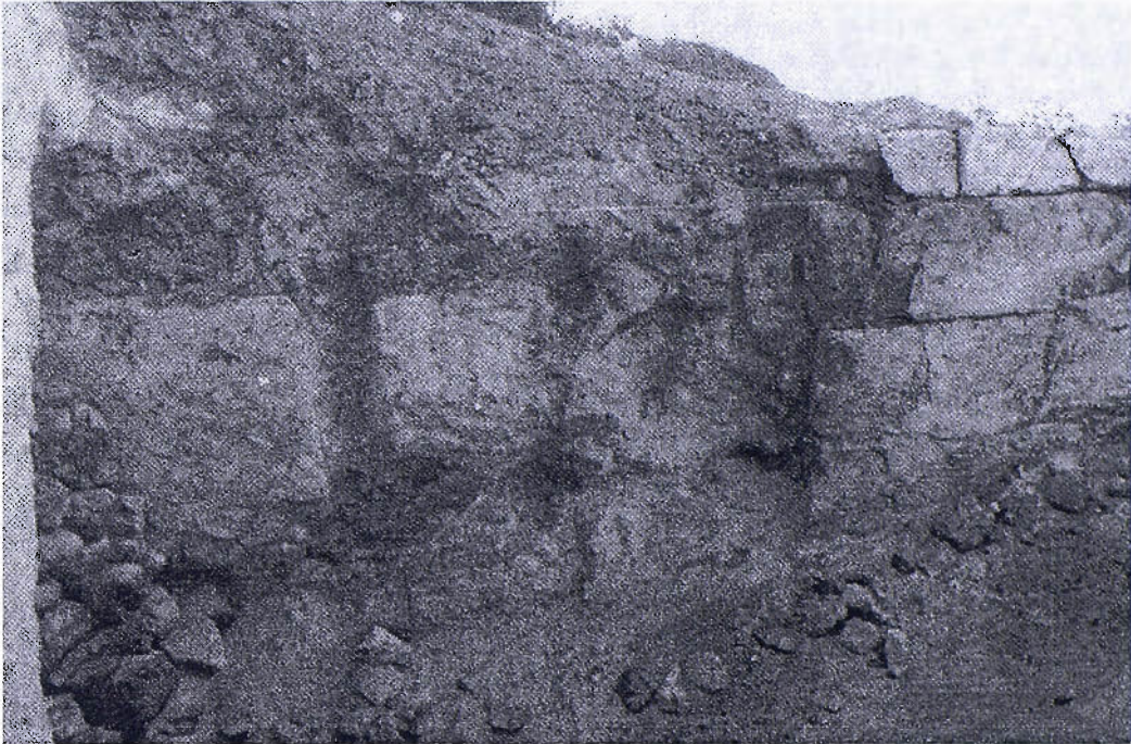
Figure 5-2: The imprint of a wooden lattice of a first floor window (Xeste 2). From the excavation archive
