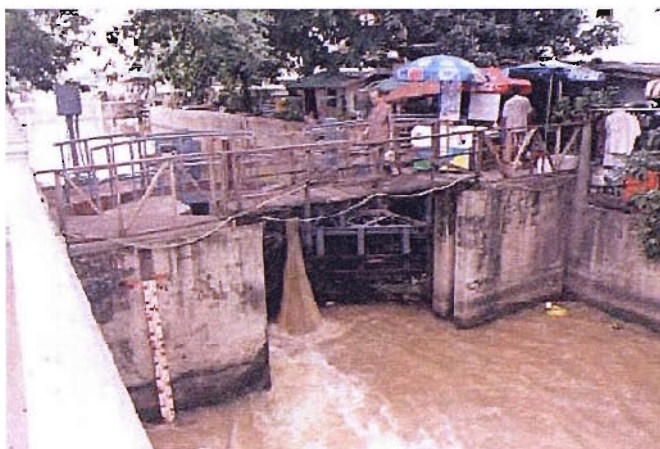
Figure 7.19: Water gate separating a city canal from the Chao Phraya River (Source: http://depts.washington.edu/agaligo/agaligo/naga/pdf/3.pdf )
