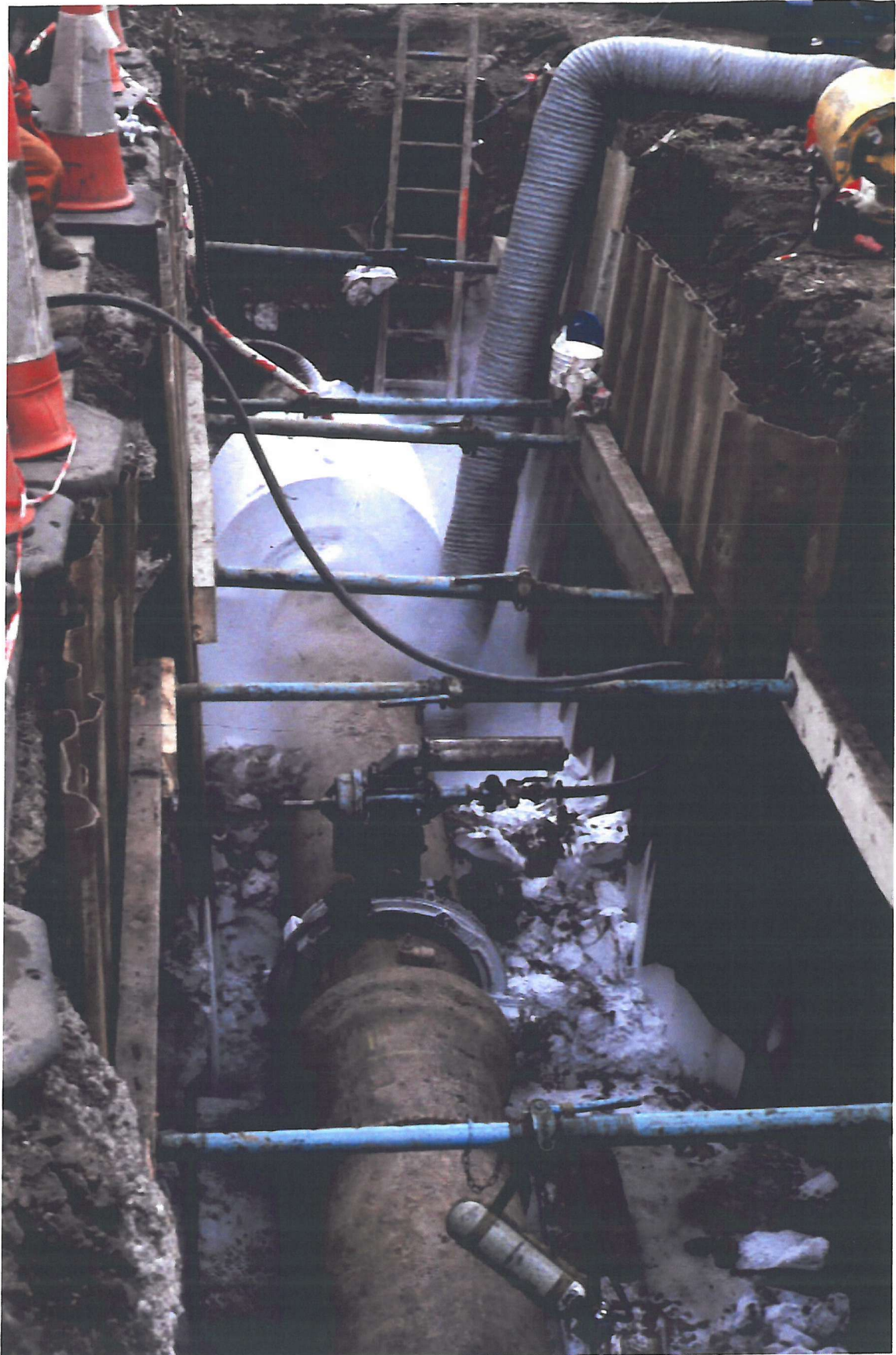
Liquid nitrogen freeze on a 51 cm (20") water main
