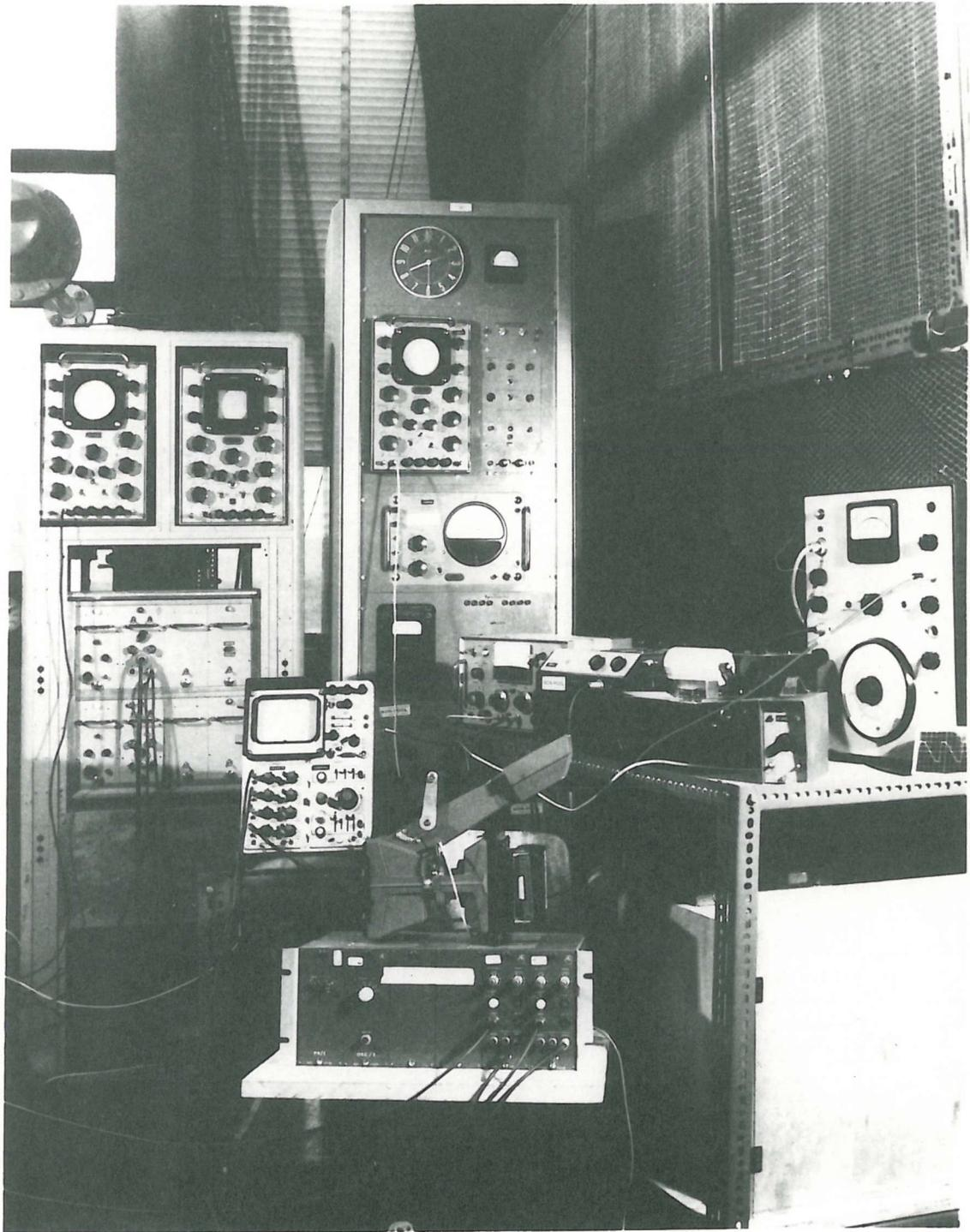
Some of the instrumentation used with the V8 Piston Slap Rig.
