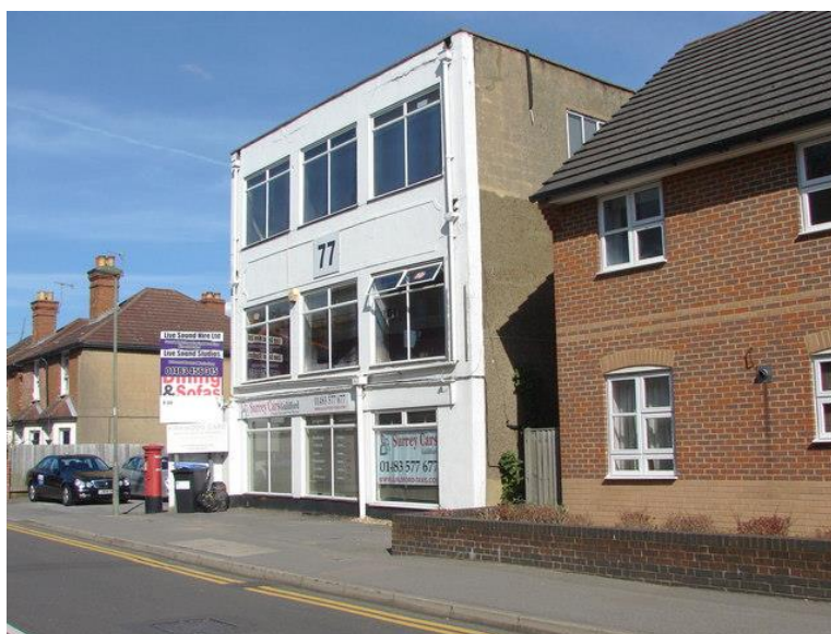
Figure 6.6 Semi-industrial buildings in Walnut Tree Close
