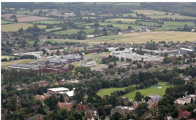
Figure 4.22 The site of QinetiQ and the Malvern Hills Science Park
