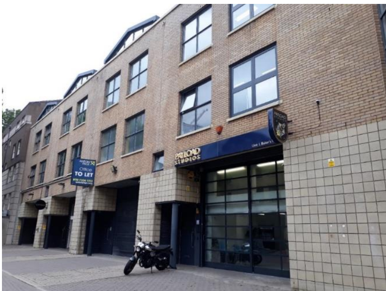
Figure 4.28 Light industrial building in Clerkenwell, home to several games companies
