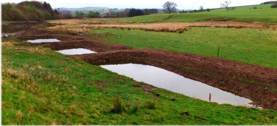
Figure 5 A sequential series of pools designed for water capture and sediment trapping for runoff from arable land from Adams et al. (2018).
