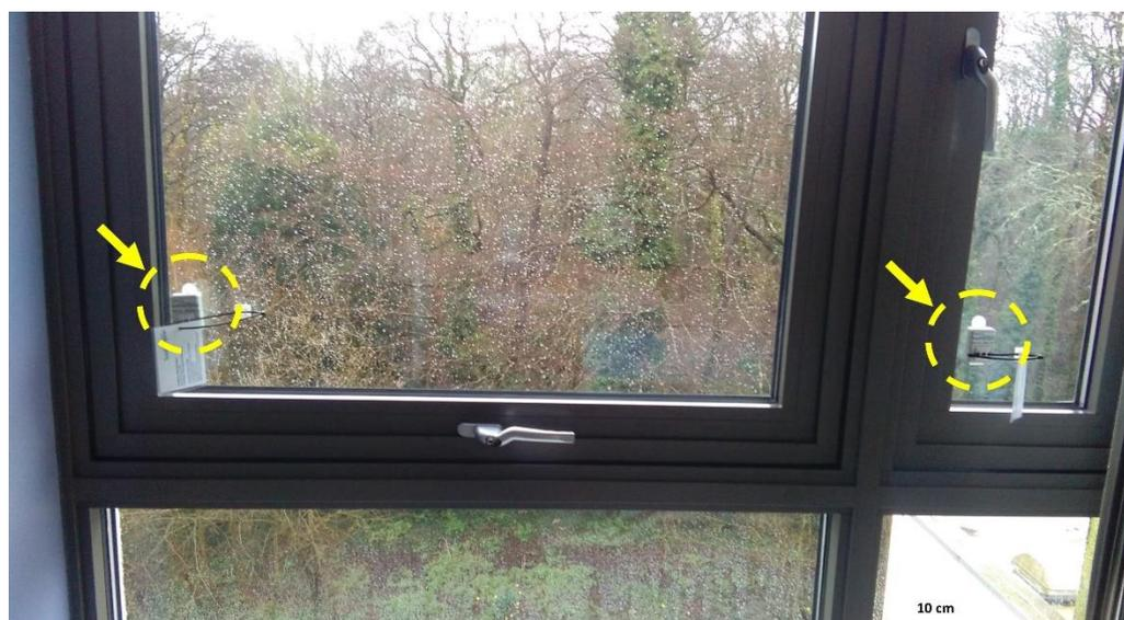
**Figure 23.** 3-axis accelerometer used to measure window movement in the control and intervention study wards during the study (1<sup>st</sup> August 2017 - 30<sup>th</sup> April 2018)
