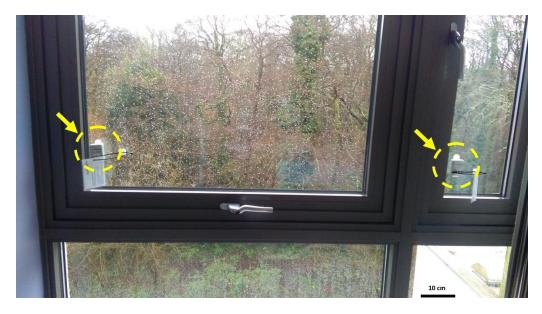
**Figure 23.** 3-axis accelerometer used to measure window movement in the control and intervention study wards during the study (1<sup>st</sup> August 2017 - 30<sup>th</sup> April 2018)
