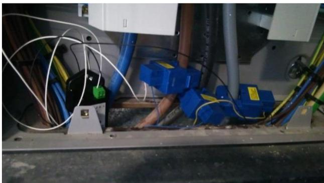
**Figure 16.** LEM AC split core current clamps and data logger used to measure small power and lighting on the electrical distribution boards for the control and intervention study wards during the study period (1<sup>st</sup> September 2017 - 30<sup>th</sup> April 2018)
