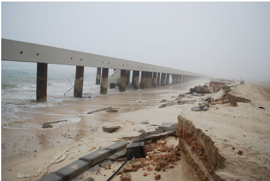
Fig. 7 Picture showing erosion off the coast of Al-Baleed near the pedestrian bridge in 2013 (taken by and used with the permission of Tom Vosmer)
