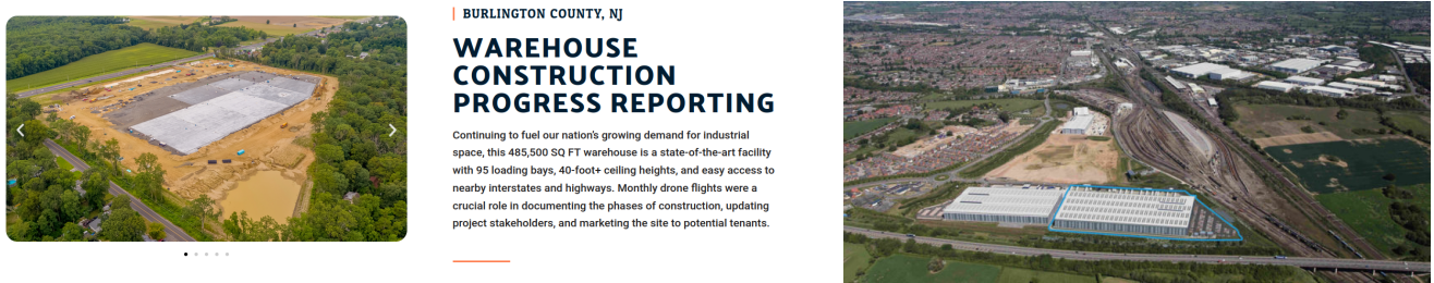
Figure 2: Left: news headline on construction monitoring (see https://thedronelifenj.com/projects/ ). Right: future projects may also consider warehouse in more crowded environments.
