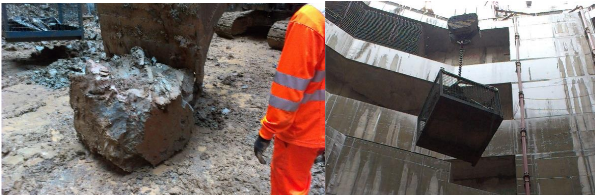
Figure 106a): Excavator trims 'lump' using fork end to the bucket b) Excavator placed 'lump' into a cage where it is craned to the surface.
