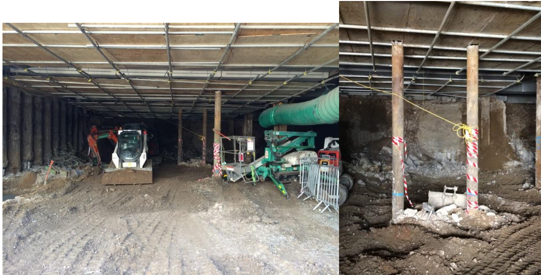
Figure 50: View of the first-floor level excavated area and the metal casings around the instrumentation boreholes, which were subsequently removed
