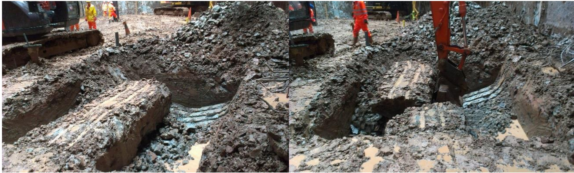
Figure 105a): Bench created by excavator at Moorgate in UMB, 40m depth b) Excavator lifts a large 'lump' from the ground by forcing forks into the sides at the base of the lump.
