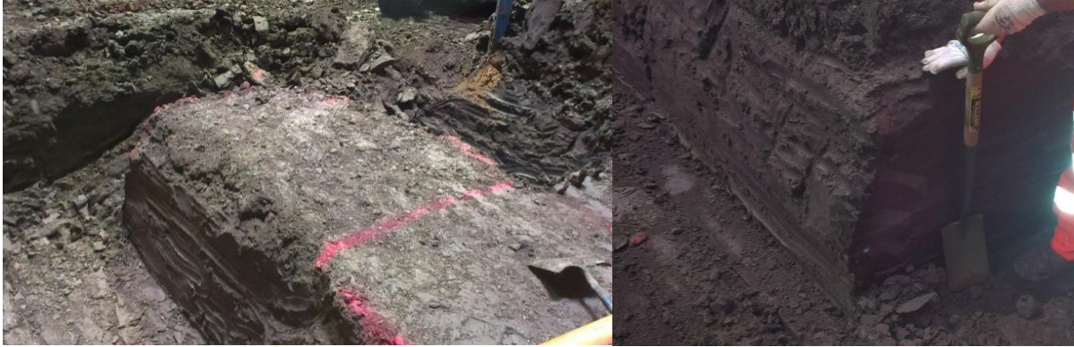
Figure 111a): Bench created by excavator at Blomfield Box in London Clay Unit A2(1) b) Shows depth of the bench
