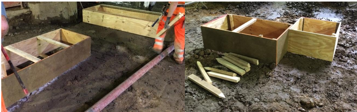
Figure 57: Formwork for the piezometers and total pressure cells
