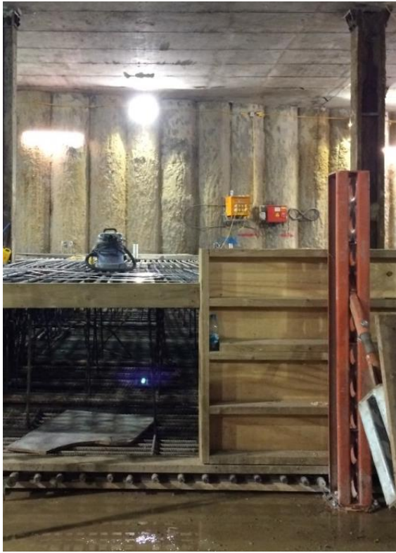
Figure 59: Formwork being built around one section of the ground-contacting basement slab reinforcement cage and the cables shown to be brought up through the reinforcement
