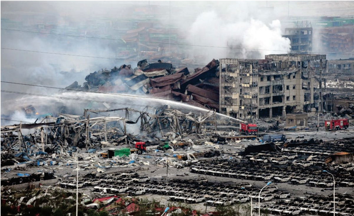
Figure 2.3: Blast damage of Port of Tianjin, China, August 2015, (The Telegraph, 2015)
