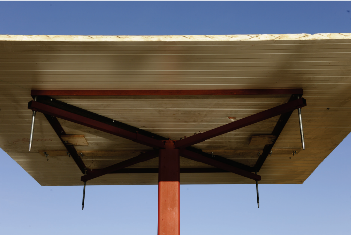
Figure 5.12: Polyurethane roof panels with steel cross-support frames.
