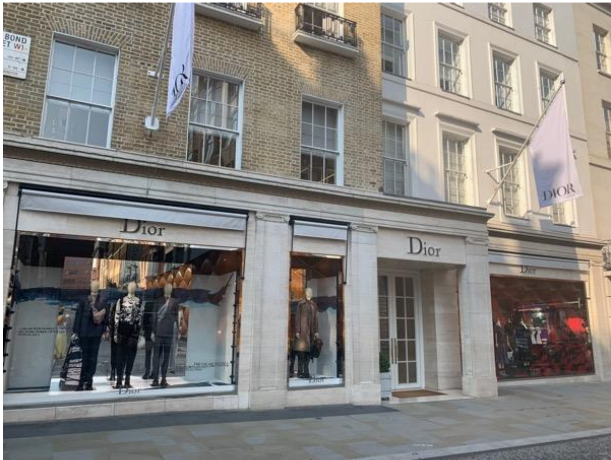
Figure 9. 22: Dior Boutique Photos, New Bond Street, London
