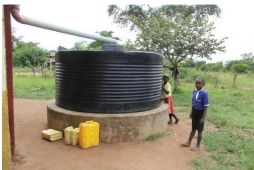
Figure 2-9: Above ground plastic storage tank (Source: Tusaidiane Uganda, n.d.)
