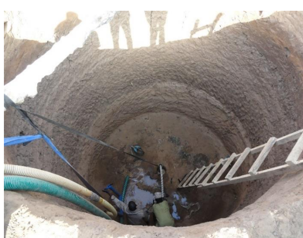
Figure 2-13: Excavation of hand dug well (Source: GWI, n.d.)
