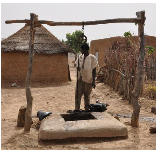
Figure 2-12: Unprotected hand dug well (Source: Appropedia, n.d.)
