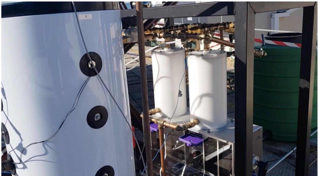
Figure 5-3 Photograph of boiler and Mk.IV condensing engine built behind the boiler cylinder on laboratory roof at the University of Stellenbosch. Reproduced with permission from Dr Michael Owen from University of Stellenbosch Solar Thermal Energy Research Group.
