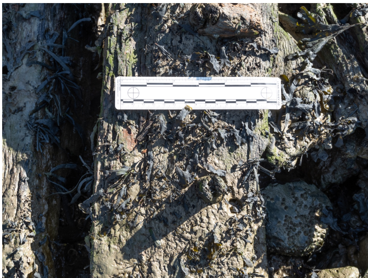
Figure 7.15: Inboard face of a treenail from Rhoda Mary showing a single wedge driven as a caulking method (Image by the Author).
