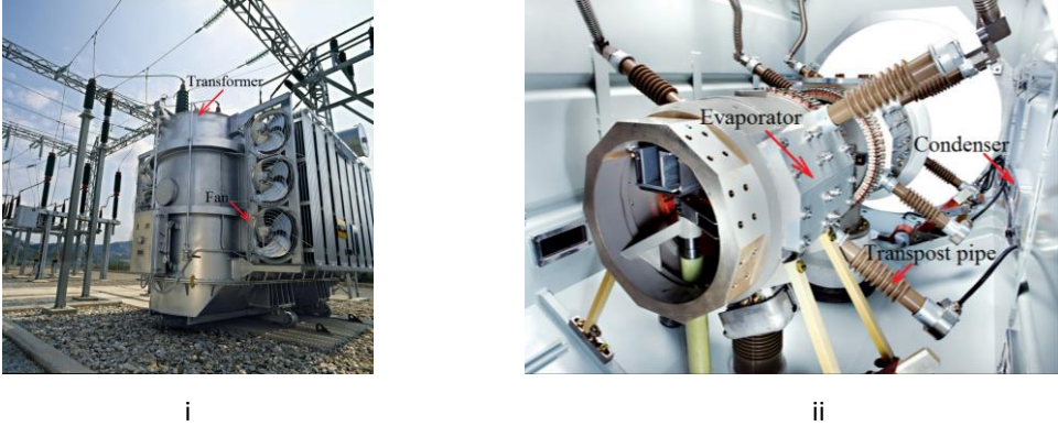
Figure 2.1 Cooling device category; i. active cooling device for a transformer, ii. Passive cooling device for generator circuit breakers
