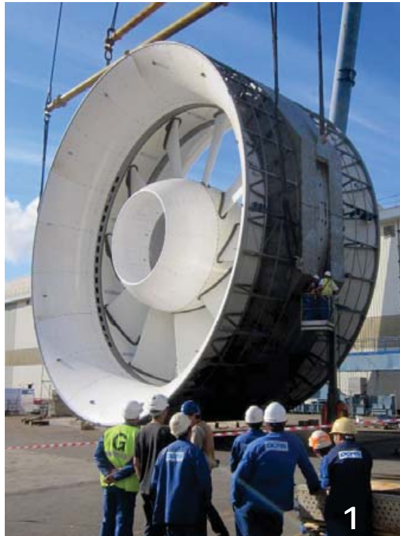
FIGURE 1.5: The 16 m prototype during construction, ©2014 IEEE.
