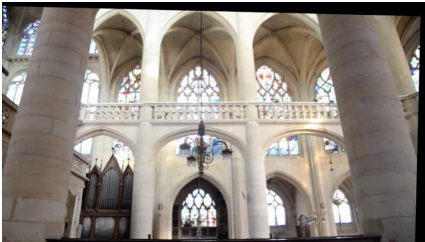
View across left side aisle
