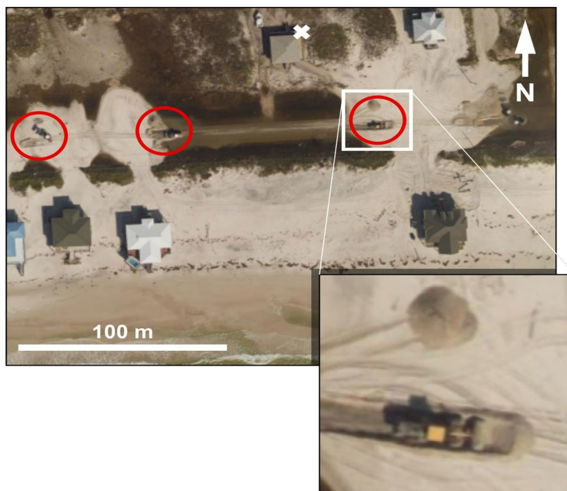
Figure 3-1 The "bulldozer" effect in action. Excavators, as circled, removing sand deposited during Hurricane Nate on Dauphin Island, Alabama, 10/10/2017 – two days after hurricane landfall (Location X: 30°15'03"N, 88°10'77"W.) Image courtesy of NOAA.
