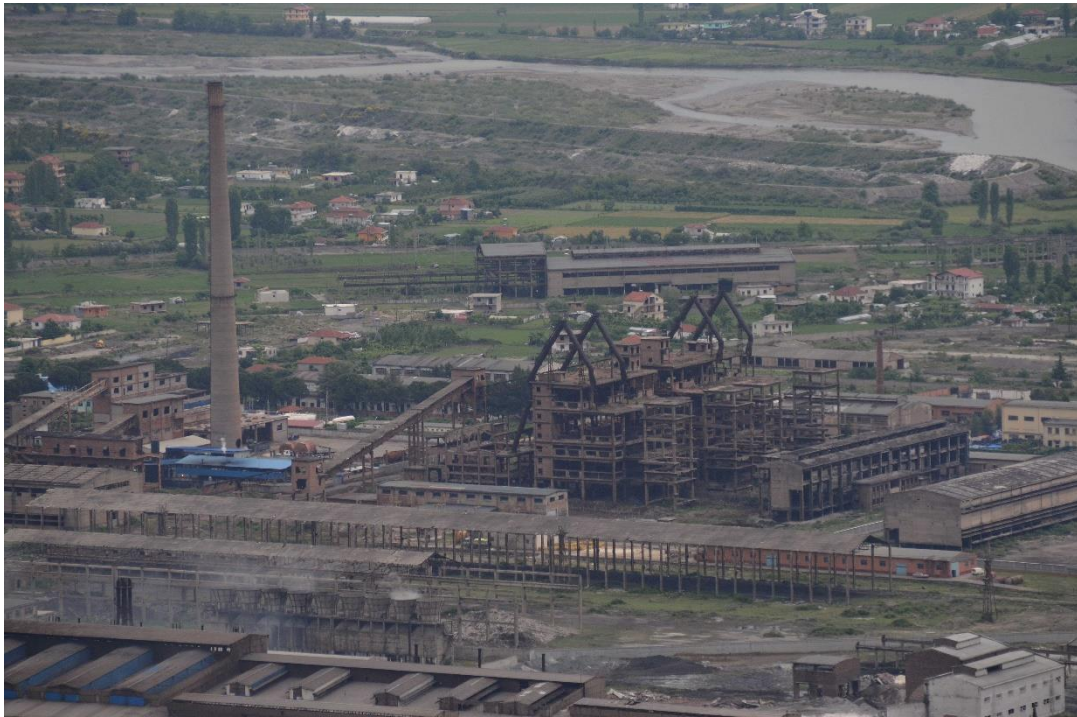
Derelict steel works, Elbasan
