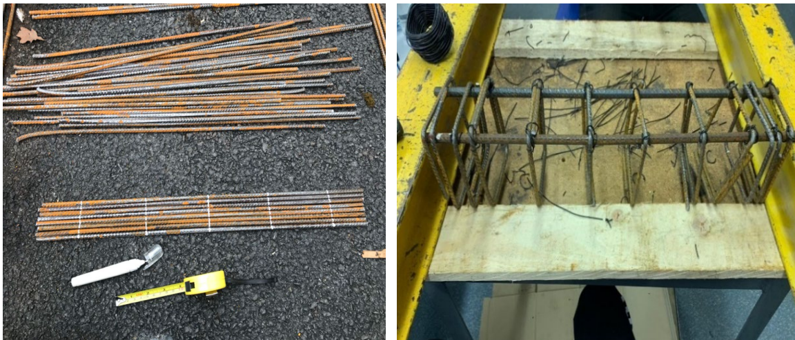
Figure 3.4: Marking, cutting and tying the rebars
