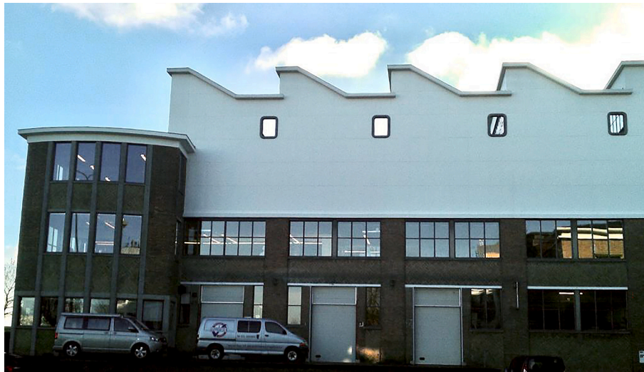
Fig. 1. Sawtooth roofs and steel framed windows (source: author).
