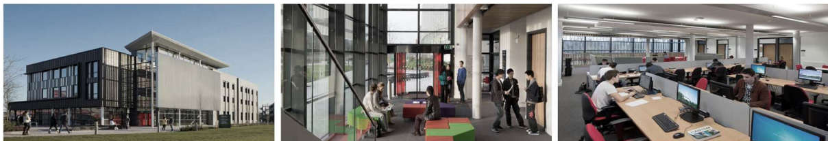
Figure 1: The exterior (left), atrium (mid) and open plan office (right) of Siyuan Centre (G F Tomlinson)
