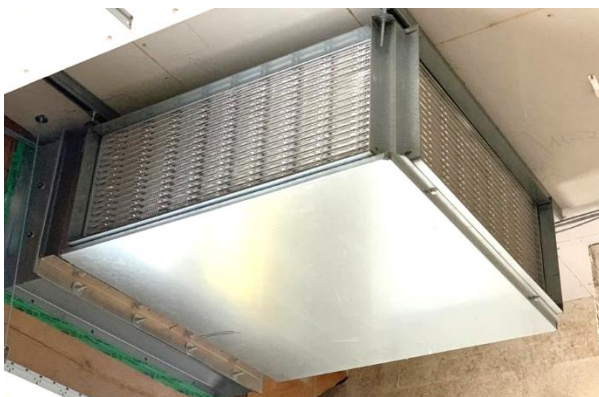
Figure 3. Crossflow plate heat exchanger, Simone Veil School, Rosny-Sous-Bois, FR (Site visit, 2023)
