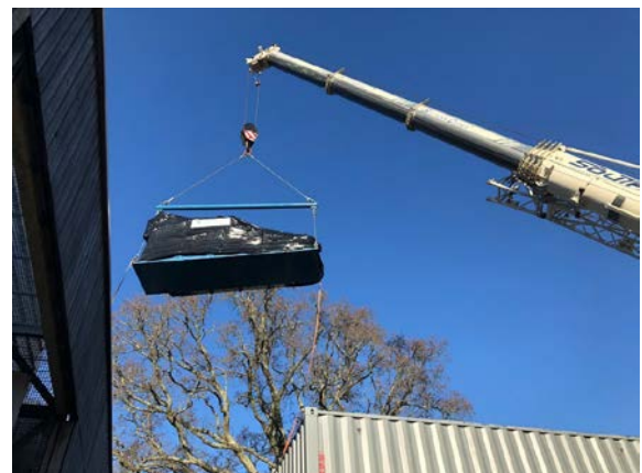
449 450 451 452 453 454 455 456 457 458 459 460 461 462 463 464 465 466 467 468 Figure 3: East winch delivery
