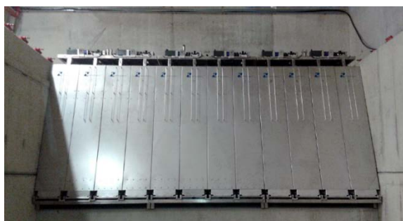
917 918 Figure 10: View of the wavemaker after installation 919
