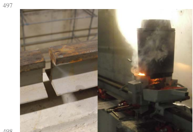
498 499 Figure 4: Rail welding
