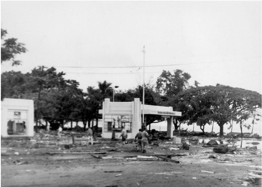
Fig. 2 Hilo in the aftermath of the April 1, 1946, tsunami in the approximate area of Bayfront Drive. Note the boulders in the foreground and the flow direction from right (seaward) to left (landward) as shown by the debris field. Photograph by Kazuo Takayama, Robynn Takayama Family Archives
