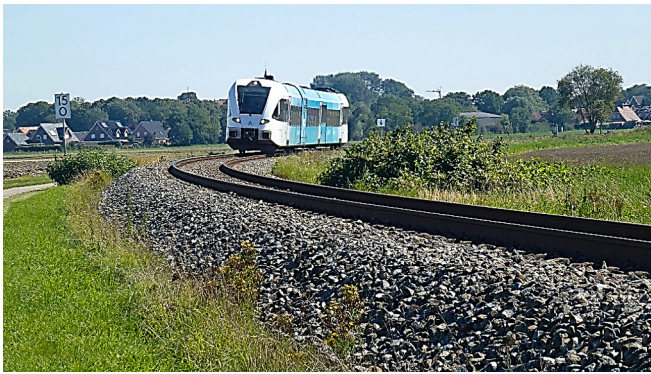
Fig. 9. Typical ballast shoulder edge slope; railway line between Bad Nieweschans, Groningen, Netherlands and Bunde, Lower Saxony, Germany. The track in the foreground is heading due west (towards the right-hand side of the picture). Date of photograph: 7 September 2023.
