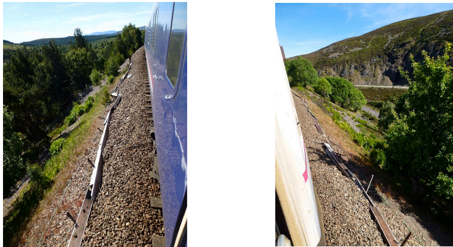
Fig. 11. Nowhere to go – the difficulty of reducing or eliminating the ballast shoulder slope; railway line near Kincaig, Badenoch and Strathspey, Scotland. The left-hand photograph is looking approximately south-west and the right-hand photograph north-east. Date: 25 June 2018.
