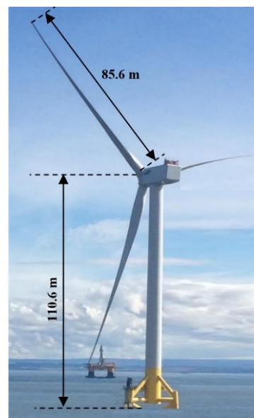
Figure 6. Main parameters and schematic of Levenmouth wind turbine [35].
