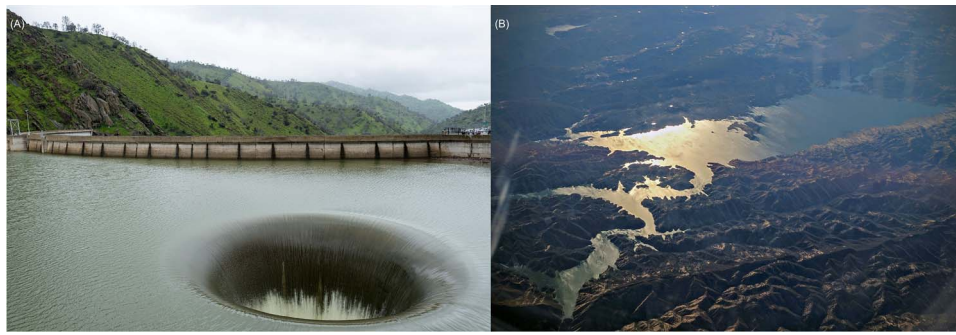
Figure 2. The “Glory Hole” spillway (A) at Lake Berryessa (B).
