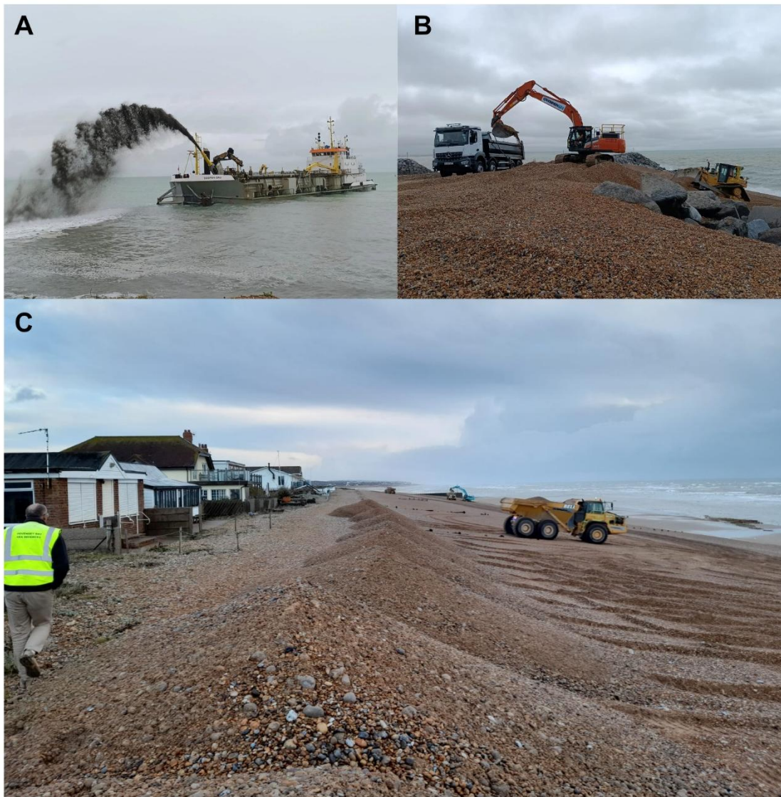
Figure 1.6 – Beach works carried out by PCDL at Pevensey Bay to maintain beach width and volume, including A) recharge (approx. 20,000 cubic m pa); B) bypassing of material from Langley Point into Pevensey Bay (approx. 8,000 cubic m pa); and C) beach recycling (approx. 90,000 cubic m pa).
