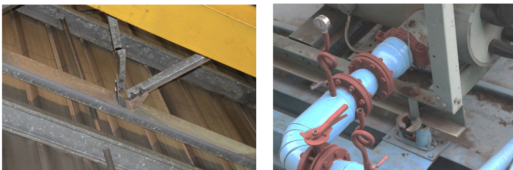
Figure 1. Examples of nonstructural elements that had bracing elements with seismic design but nevertheless experienced failure during an earthquake (Photos by Eduardo Miranda).
