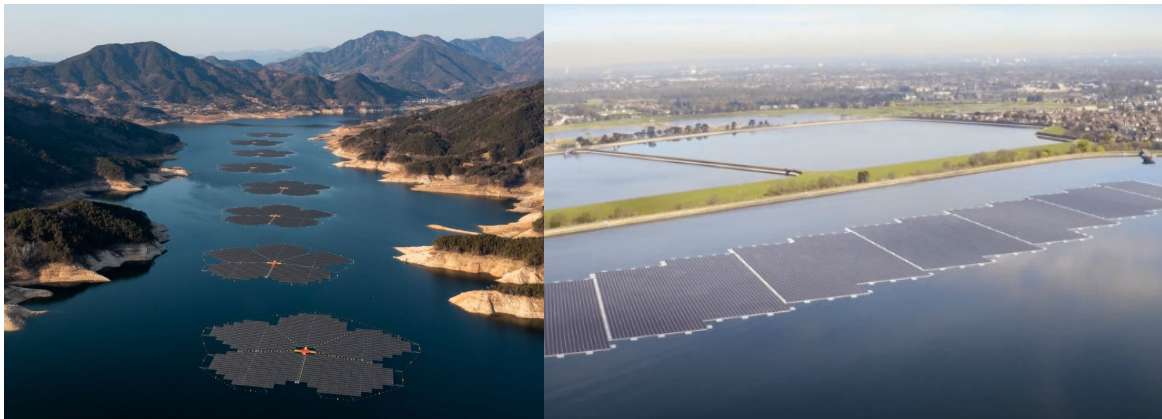
Figure 8-50. Floating solar panels on the surface of the Hapcheon Dam in South Korea (40.32 MW) and Queen Elizabeth II Reservoir floating solar (6.3 MW) [170, 171]
