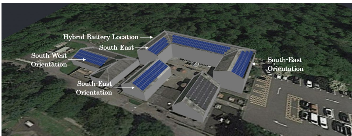
Figure 8-54. Roof mounted PV, Hybrid Battery Storage, Dare Valley Country Park Hotel
