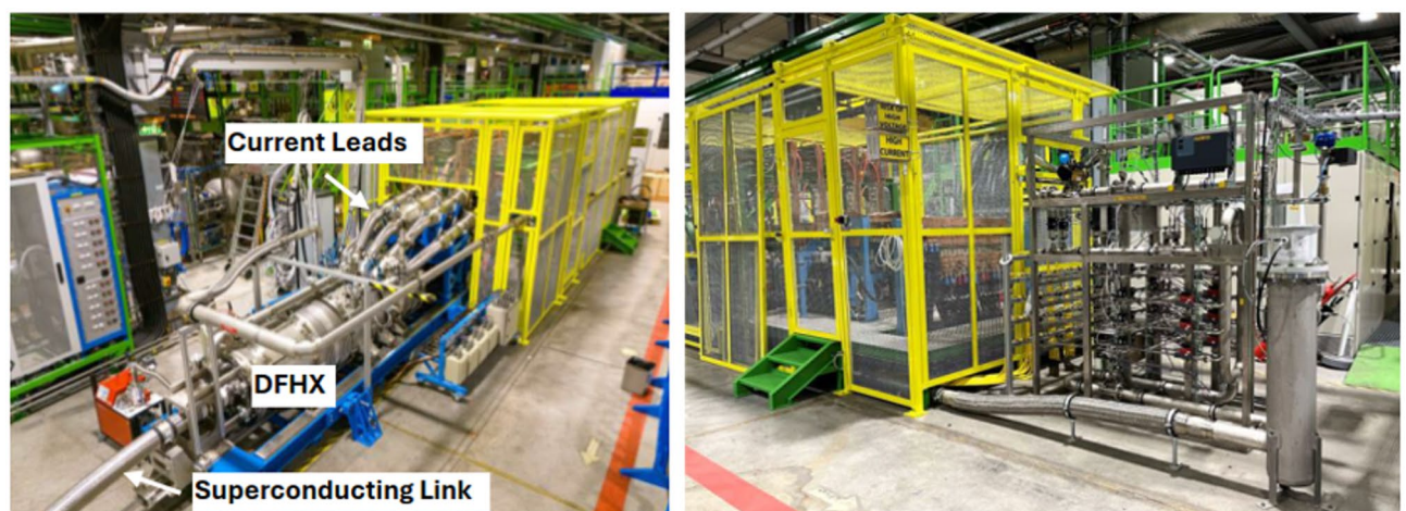
Fig. 5. DFHX and room temperature cables inside the IP2X yellow cage. Gas management system in front of the IP2X yellow cage with the room temperature cables distributed and connected to the current leads. It contains helium valves and helium gas recovery lines.
