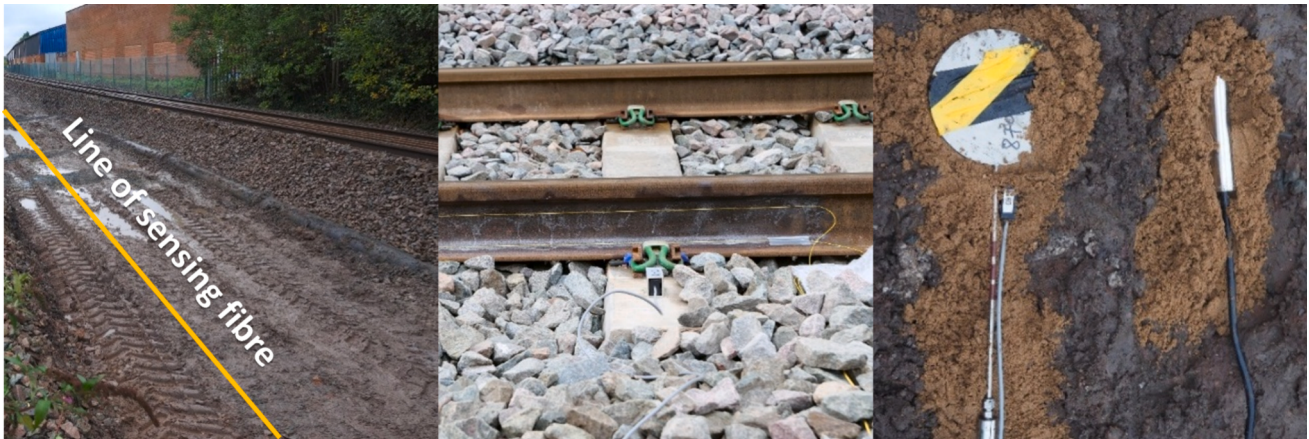
Fig. 2. Site 1 (a) buried fibre, (b) final installation (c) buried instrumentation.
