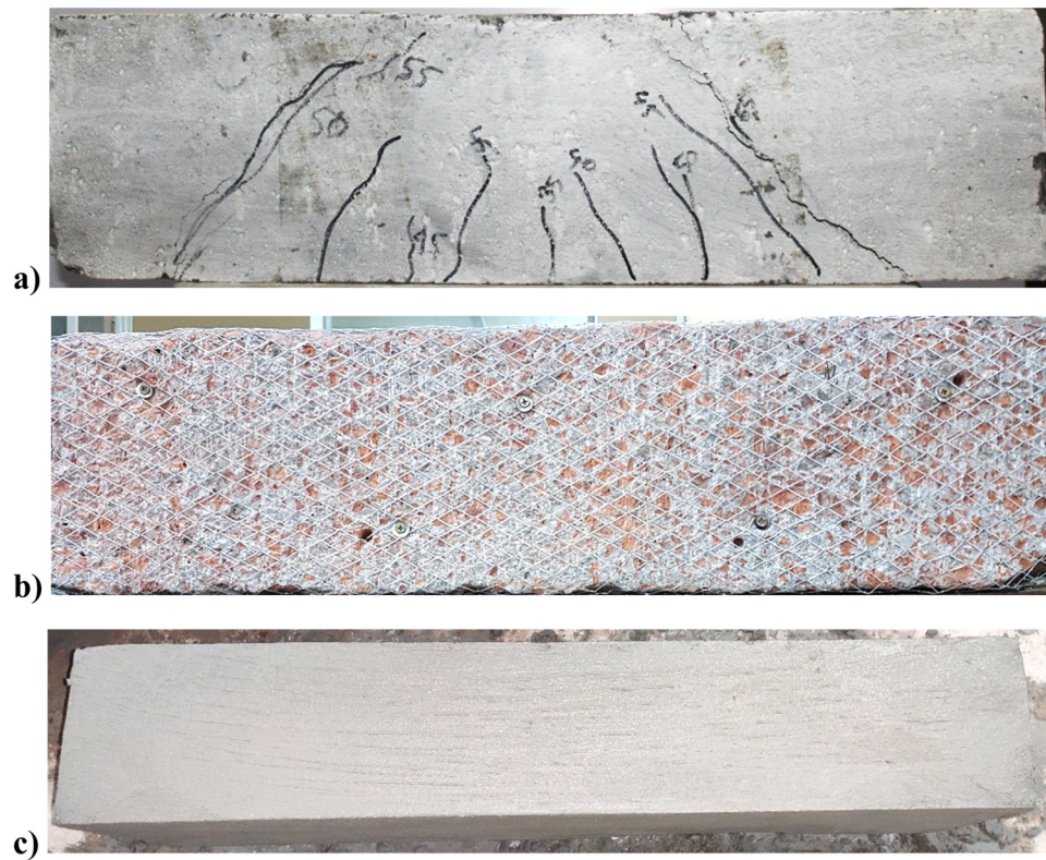
Fig. 4. Strengthening of beams utilising the ferrocement method: (a) damaged the beam nearly collapsed, (b) roughening the strengthened surface of the beams and wrapped with steel wire mesh U-shape jacketing, and (c) application of cement-based mortar on the beam surfaces.
