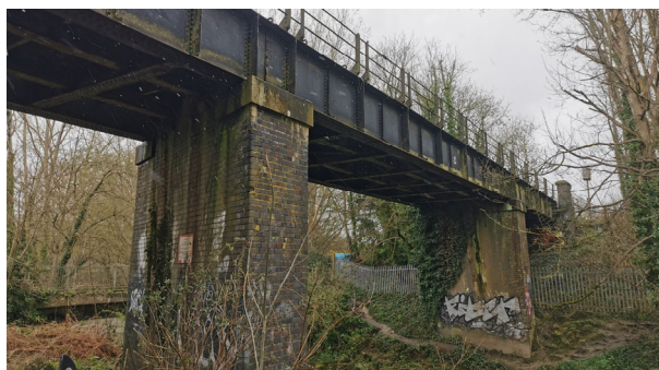
235 236 Figure 2: Upside elevation of the three-span, single track, half-through type, early steel railway 237 bridge examined as a case study.
