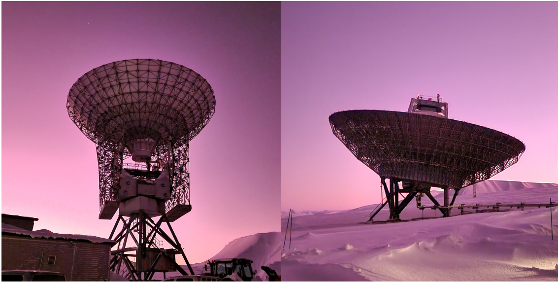
Figure 3.17: The 32m (left) and 42m (right) parabolic dish antennae of the ESR, with red sky enigma.
