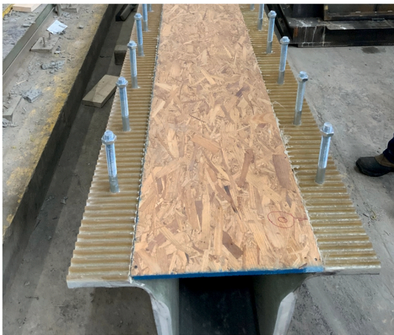
Fig. 4. Photograph of the glass-carbon FRP composite girder before concrete casting.
