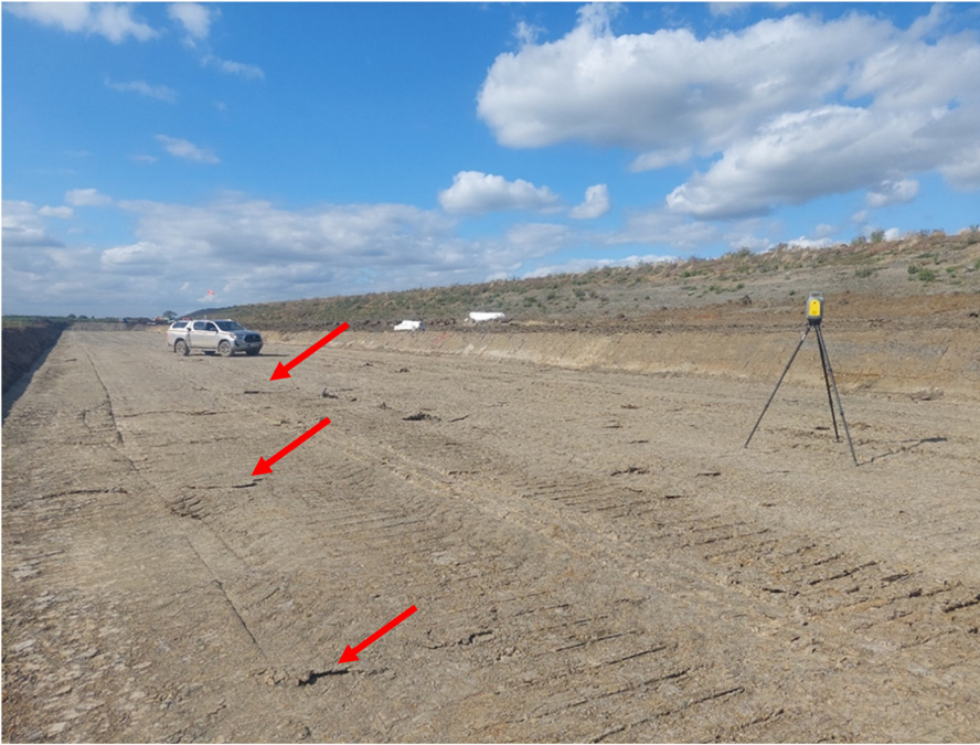
Fig. 10. The base of a 2 m excavation near Waddesdon (WA), Buckinghamshire. Some deeper shear surfaces are evident over a 40 m length after initial proof rolling with a vibrating roller.
