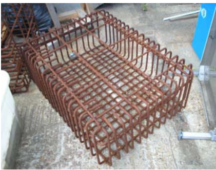
Fig. 4 Typical Reinforcement Cage
